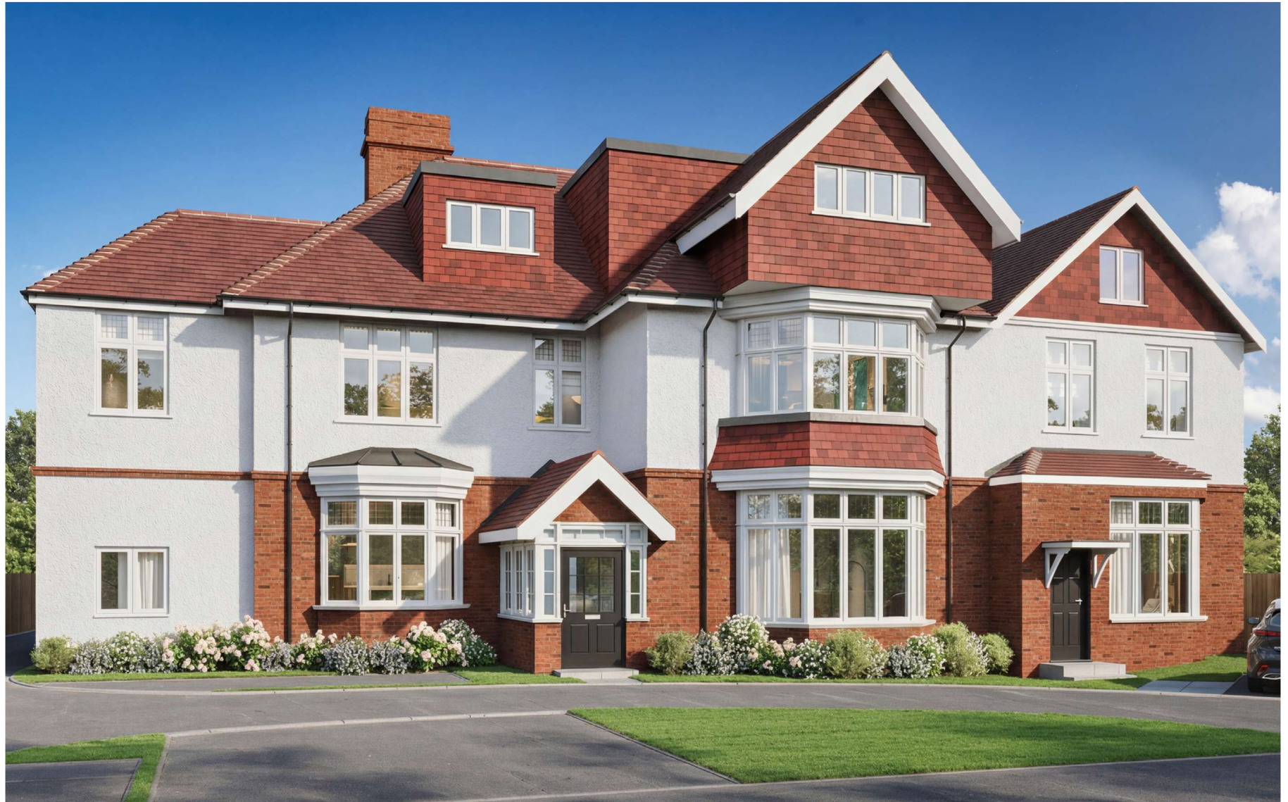
FLATS 1-7 GRANTLEY COURT — VIEW FROM YORK ROAD
